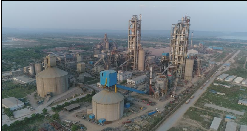
Cement Plant Project, Rajasthan
