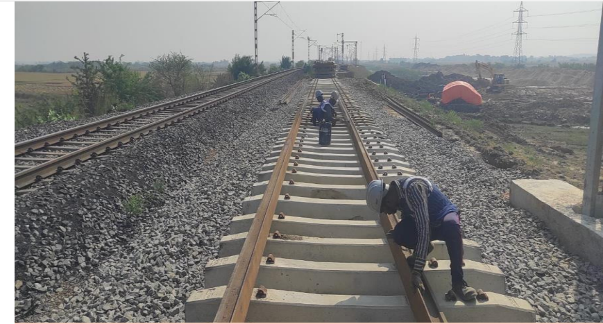
Railway line for Port Connectivity project in Dhamra, Odisha
